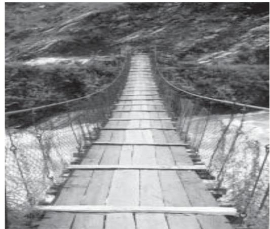
*Wooden walkway deck need changing every three to four years. Galvanized steel walkway deck is relatively 'maintenance-free'*
