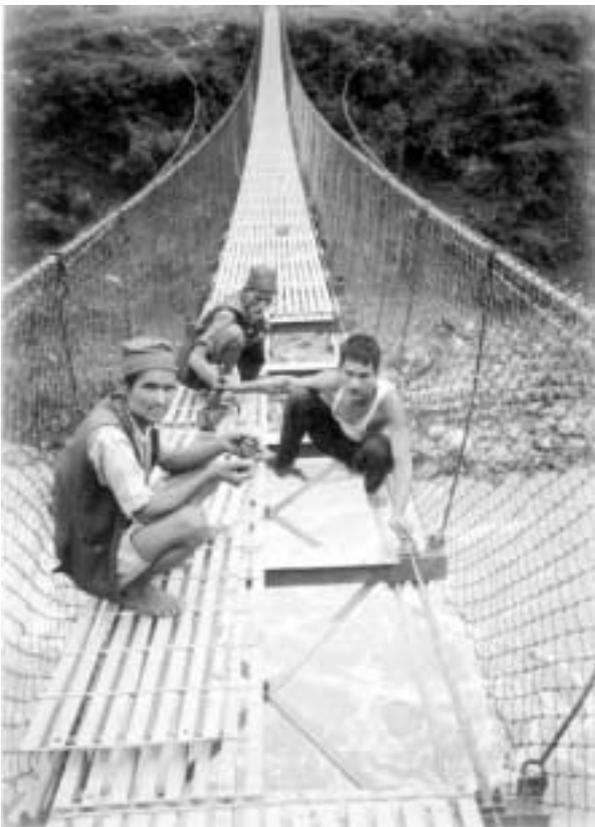
*Major maintenance work: wooden decks of old bridges are replaced with steel decks*
