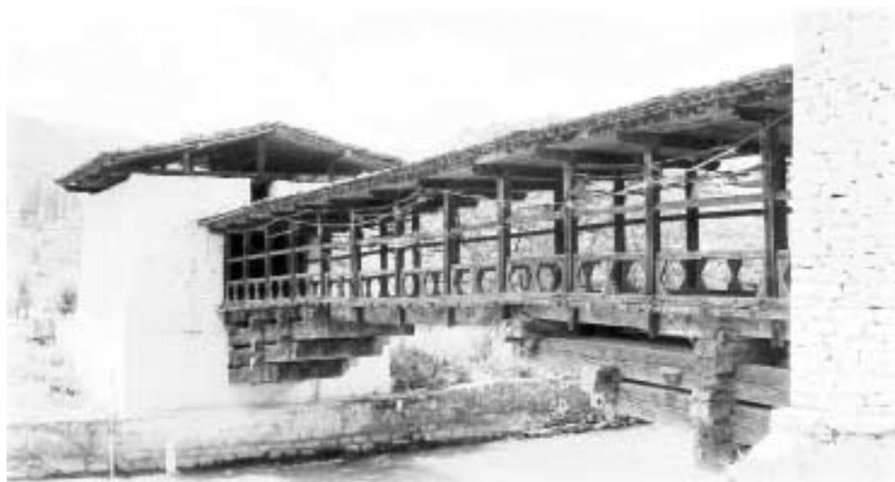
*A traditional Bazaam bridge - roofed wooden cantilever bridge, Bhutan*
